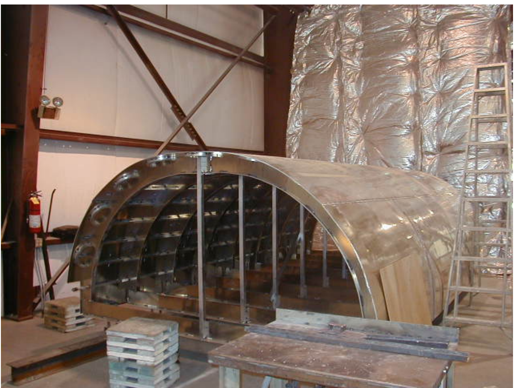
Mold for the cylindrical house
