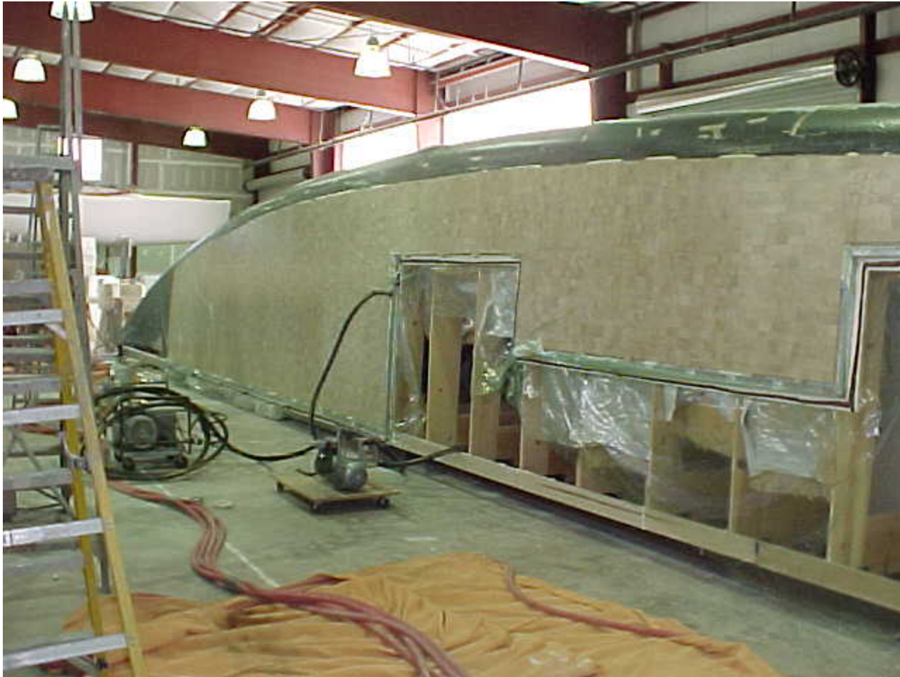
Vacuum bagging the SuperLite Balsa core
